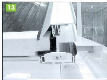
Fit the starter bar top capping into position.
