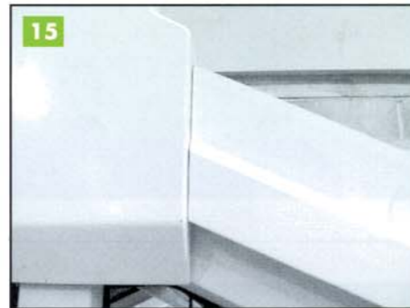
Offer the lean to cloaking trim up to the side of the gable ridge end cap and scribe to suit the roof pitch - push into place against, the end cap.
