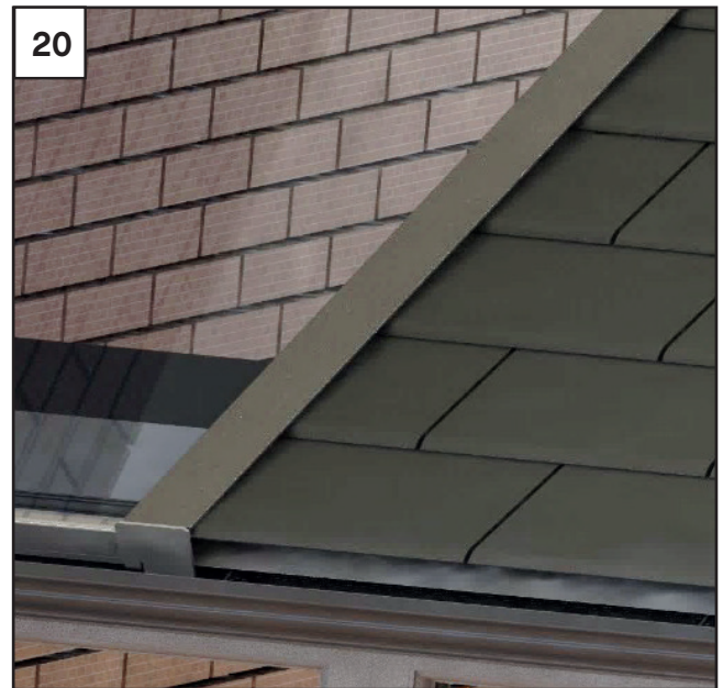
Tile rest of roof. Leave approx. 20mm gap between end of tiles and soaker rail upstand to allow glazing bar top cap fit. Push glazing bar top cap down securely into PVC Thermal break, ensuring even seal on the gasket onto the glass. Expanding foam seal should expand to fill voids against the tiles.
